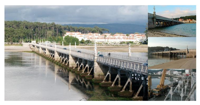
The new La Toja Bridge replaces a bridge which was completed in 1915 and which was one of the first reinforced concrete bridges in Spain. Its substitution became inevitable due to increasing problems of durability that had been affecting the structure from the beginning.
